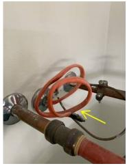
**Photo 27-1** Electrical wire for a electric water heater.
